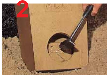
2 Drill out/cutout holes for pipe connection.
