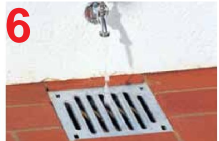
6 Ensure finished surface is 1/8" higher than the grate to assist water drainage.
