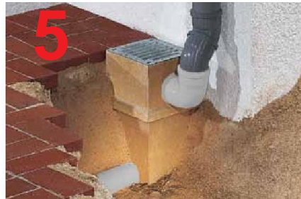
5 Add riser (if required) and connect inlet pipe (if required). Surround PointDrain with good quality concrete. Finish with surfacing material.
