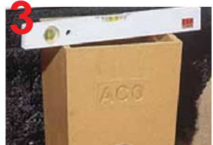
3 Position PointDrain on a 4" thick concrete slurry bed and ensure it is level.
